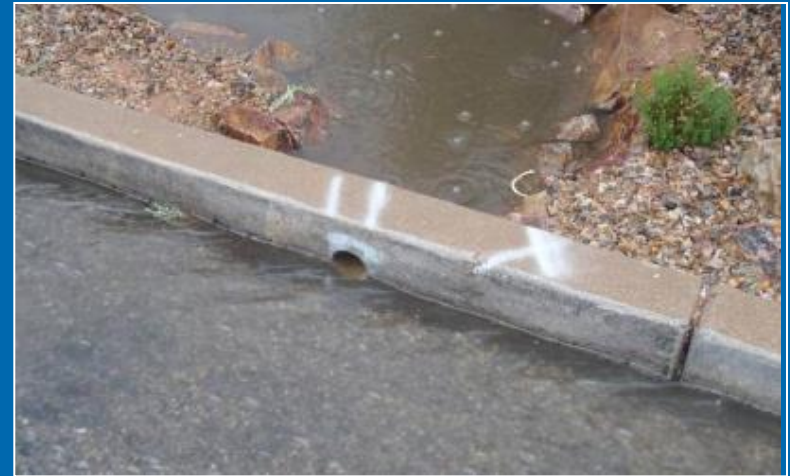
Curb Core for Street Run-off
