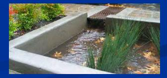
LID "Toolkits" from an **Engineers** Perspective LID is a requirement of NPDES permit (AZ) City of Glendale / City of Mesa LID toolkit In use, must assume capacity of system will be exceed for all swales, basins, curb cuts, bio retention! In arid SW, still requires additional water sources such as irrigation Maintenance of LID item (ROW / Private?) Engineer – function is most important! Flow control, detention, retention, filtration, infiltration, treatment – DUST WILL accumulate !!!!
