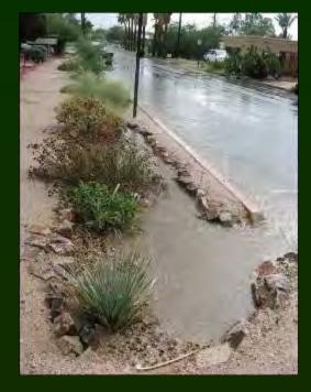
Old design: water collects, causing pavement failure
