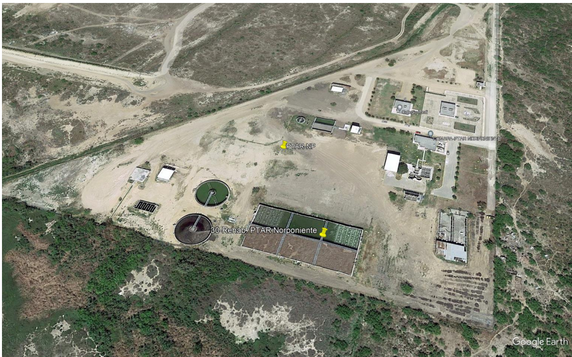
Figure 5 NORTHWEST WASTEWATER TREATMENT PLANT
