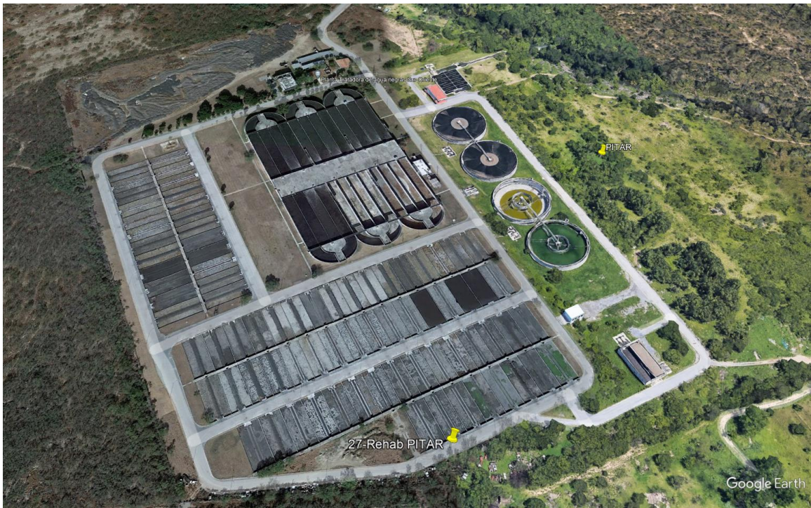
Figure 4 INTERNATIONAL WASTEWATER TREATMENT PLANT
